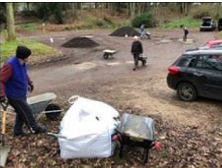
Exhausting work for our volunteers spreading 20 tons of road planings
